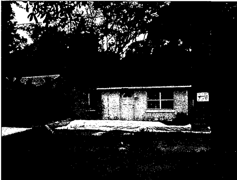
Single-family home for clergy, 4723 Pinedale Avenue
